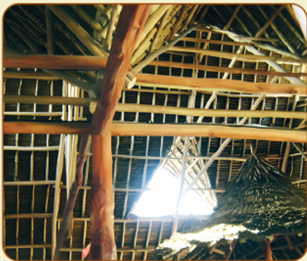
Casuarina poles for roof construction
