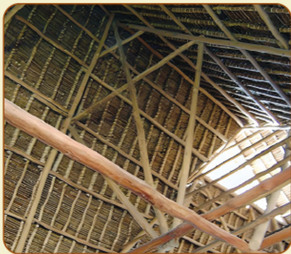
Casuarina poles for roof construction
